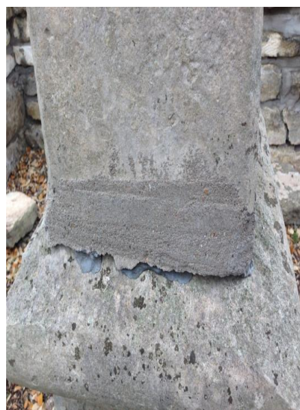
Figure 6: Modern materials used in restoration
