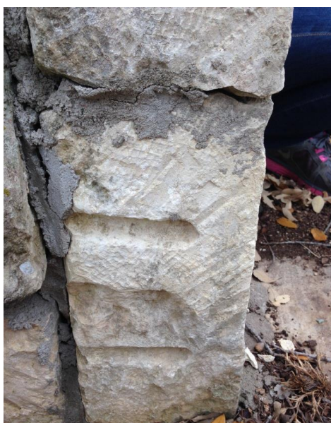
Figure 7: Reversed gate hinge block
