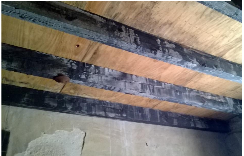
Figure 4: Burnt beams of first floor ceiling in living room.
